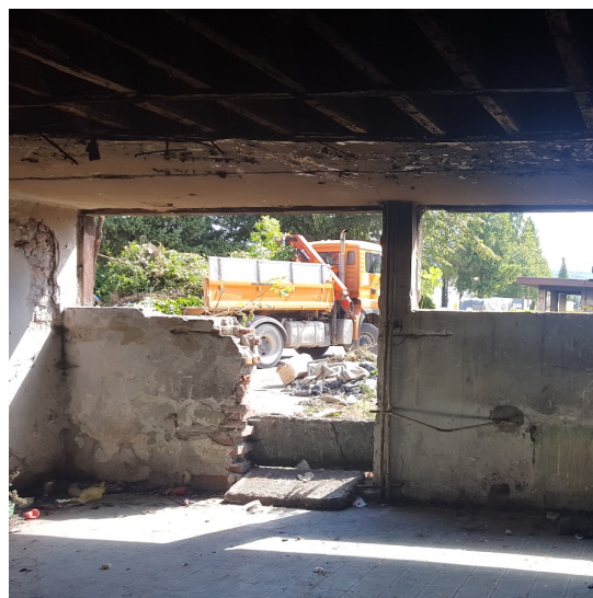
Squat being cleared and cordoned off (Source: BVMN )
